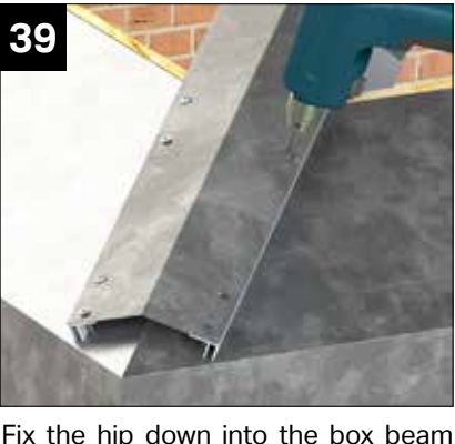
Fix the hip down into the box beam through 4 x pre-drilled holes using WPCS020 screws (provided). NOTE: The external box beam cleat is still required.
