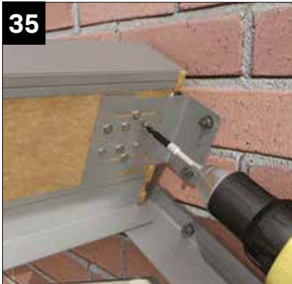
Finally secure the rear ridge fixing bracket using 8 x NRTF050 (PROVIDED) one bracket on each side of the ridge.
