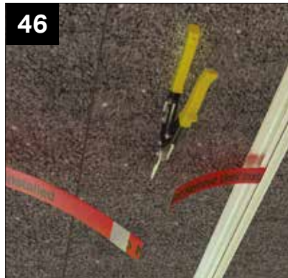
When in position snip the retaining straps. Straps might be red or black.
