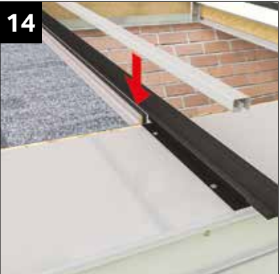
The external half clip being installed (see solid roof section for fitting of external and internal panel clips).
