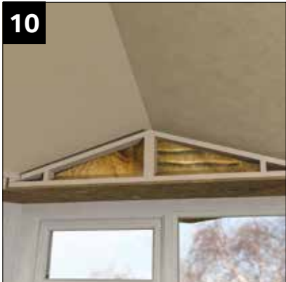
10 Insulate void with mineral wool.
