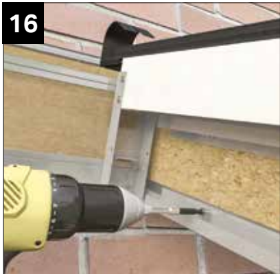
Then fix the lower 'U' channel.
