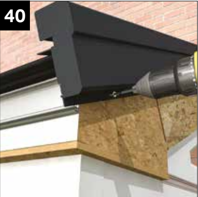
Fix the dry verge to the OSB using NRTS 050 screws at 300mm centres. Ensure membrane overlaps into dry verge for drainage.
