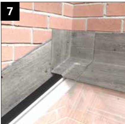
Finally, manipulate code 4 lead over the glazing bar top capping and half ridge capping with overlaps as step 31 page 55.
