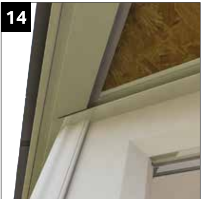
14 External ship lap cladding edge channel detail.
