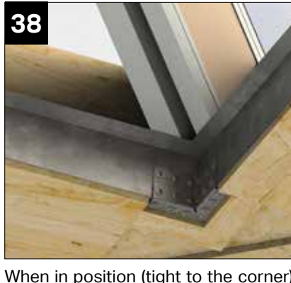
When in position (tight to the corner) the hip should sit on the box beam shelves.
