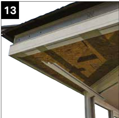
13 Fit external ship lap cladding edge channel.
