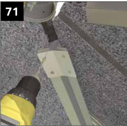
Fix the internal upper hip brace plate using 4 x CHAA 006 screws provided. NOTE: These plates are not required on victorian hips.
