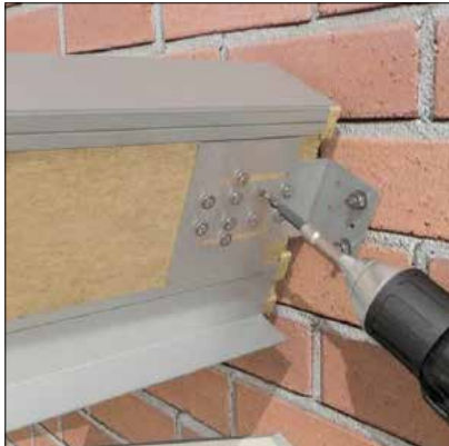
Finally secure the rear ridge fixing bracket using 8xNRTF050 (PROVIDED) one bracket on each side of the ridge.
