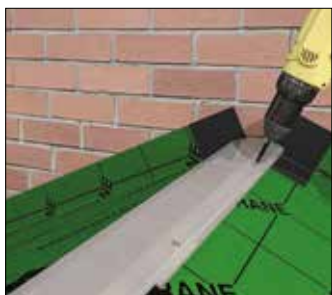
Fixing ridge under capping into tile stop 500mm CTRS
