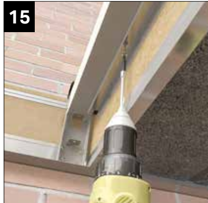
To secure the glazing bar offer the upper 'U' channel section. Screw up through into the bar within 200mm of the wall plate and box beam. Then at 500 centres. Using NRTS050 4.2 X 25mm screws provided. Then fix horizontally into OSB at similar centres.
