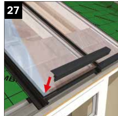
Prior to fitting the pre-notched glazing end profile, run a bead of silicone, low modulus (for non coated glass) or MS polymer (self cleaning glass) immediately behind, the co-extruded gasket before tapping down into position. Then seal each end to protect the seal.
