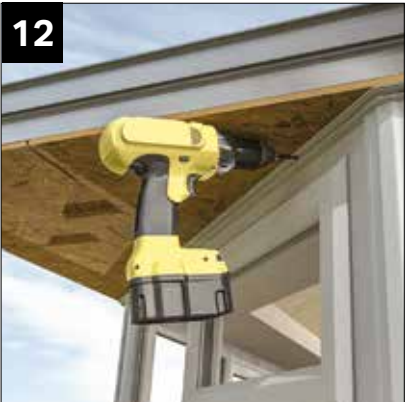
12 Fit external soffit channeling.
