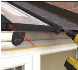
Fixing glazing bar end caps Pre drilled holes
