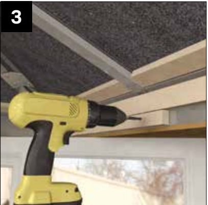
3 Attach additional battens.
