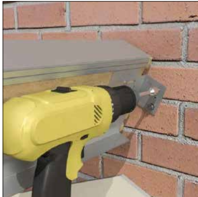
Reposition ridge and secure to the host wall using resin anchors suitable for substrate (NOT PROVIDED).
