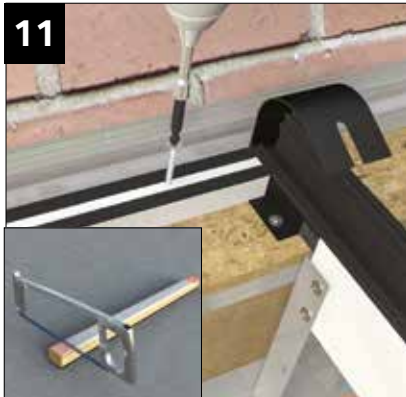
Turn the upper wall plate glazing support trim upside down and cut small notch into each end to allow support trim to sit flat onto the OSB board and tight into the bars. Secure the upper wall plate glazing support trim using 2 x WPDS 020 3.5 x 50mm screws provided.
