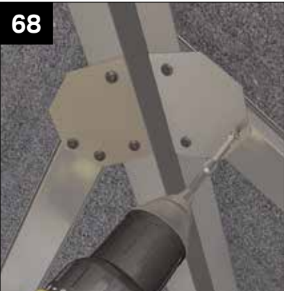
Where jack rafter abuts hip bar fix the jack rafter connection plates using 4 x CHAA 006 screws provided. NOTE: fit one screw through half clip that meets hip bar.
