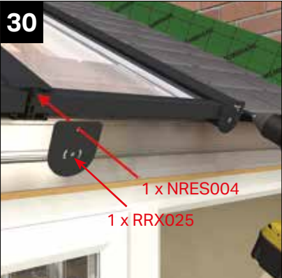
Attach the transom end cap plate to the end of each glazing bar using • Top screw - 1 x NRES004 • Bottom screw - 1 x RRX025 Screws are provided and each screw has 2-part coloured cap cover.
