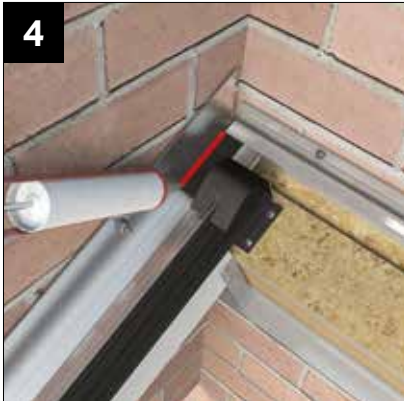
Silicone the edge of the bung against the starter bar.
