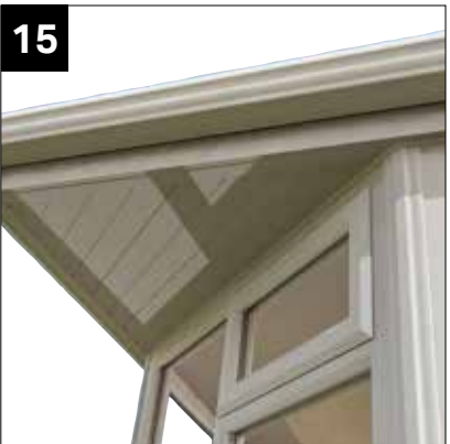
15 Cut and fit ship lap to suit.
