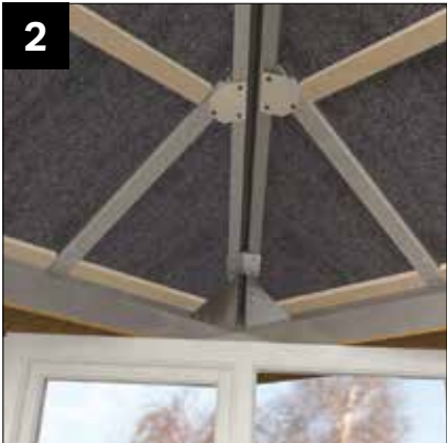
2 Batten out to suit plasterboard fixing.
