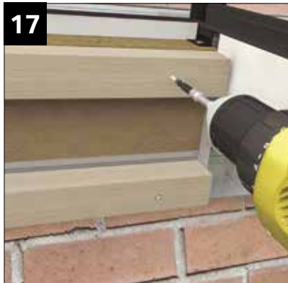
At the wall plate fix the upper and lower plaster board timber battens (45 x 45mm) with screws (not provided) one fixing either end. The upper timber finishes flush with OSB board.
