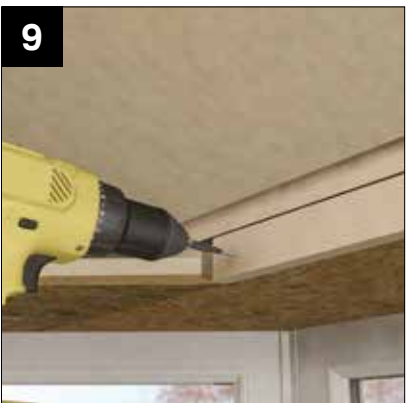
9 Attach additional mating timber battens.
