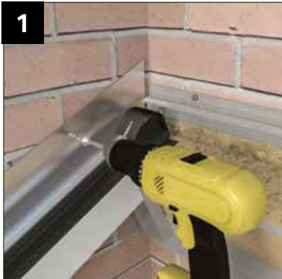
Set the half ridge (wallplate) 5mm away from the host wall. The height (as step 6 page 47). Upper end of starter bar positioned so that glazing gasket aligns with glazing support trim. Secure to host wall within 200mm of half ridge and box beam plus at least one more equidistant between the two. Use resin anchors suitable to substrate - not provided.
