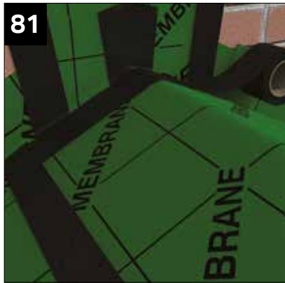
Use tape to seal the layer at ridge end.
