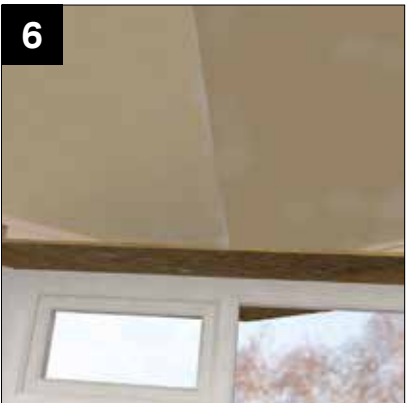
6 Plasterboard the roof.
