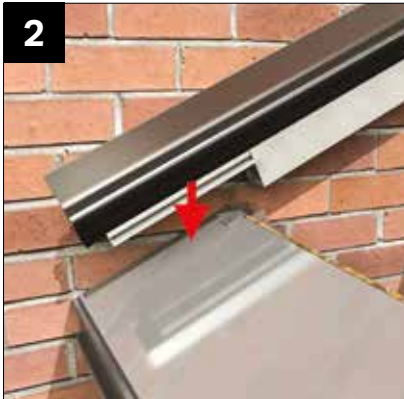
Starter bar rides over the front box beam and drops into box beam shoe. Secure the shoe with 2 x (NRTS 050) screws.
