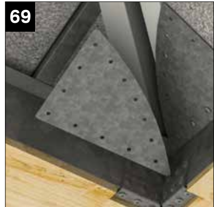
Fix the internal hip retaining plates using 18 x CHAA 006 screws provided into the box beam shelf and hip bar. NOTE: These plates are not required on victorian hips.
