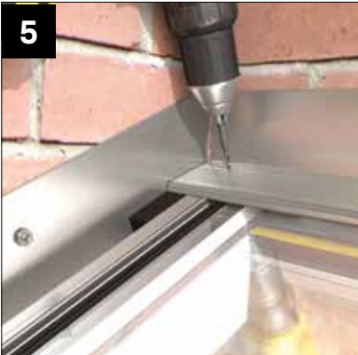
Secure the half ridge top capping into starter using (CHAA006) screws provided.
