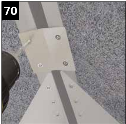
Fix the internal lower hip brace plate using 4 x CHAA 006 screws provided. NOTE: These plates are not required on victorian hips.
