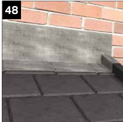
Lead flash to exiting host wall.
