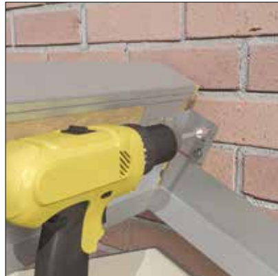
Once ridge is set and level, drill through brackets into host wall, THEN REMOVE SETOUT COMPONENTS.
