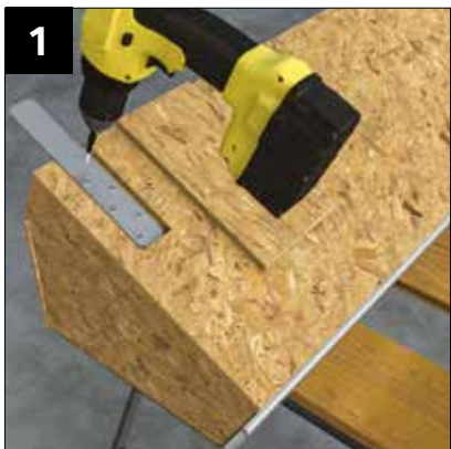
Fix the aluminium gable beam fixing plate to the underside of the box beam using 6 x RRR 025 screws. NOTE: ALIGN PLATE 'V' NOTCH GROOVES WITH EDGE OF BEAM.
