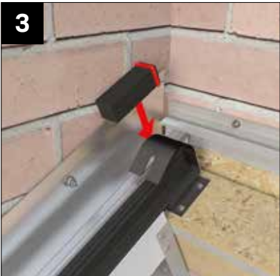
Seal top edge of starter bar bung (NRTA002). Place the bung tight into the junction of the host wall and starter bar. Then seal with clear low modulus silicone.
