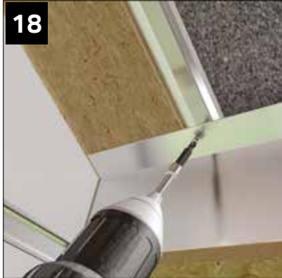
Secure the gable end panel (s) only by screwing up through the box beam shelf and the upper half ridge shelf using 1 x NRTS050 screws provided.
