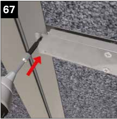
Secure attachment plate using 2 x CHAA 006 screws provided to the ridge body.
