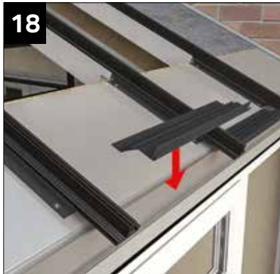
At the box beam end of the glazing panel, locate aluminium glazing support trim between glazing bars. See inset at step 19 for location point.
