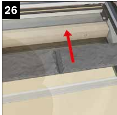
Slide into position the half ridge tile screen. This will be trapped into position when plaster boarded. See separate tiling guide for details of tiling method.
