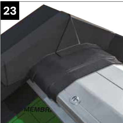
Finally cover joint with a third layer.
