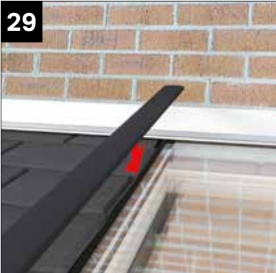
Finally knock on the aluminium glazing bar top capping. NOTE: Ensure to check the brush seal runs down tiles and Q-lon gasket runs down the glass. Angled end of capping to half ridge, square end at box beam end.
