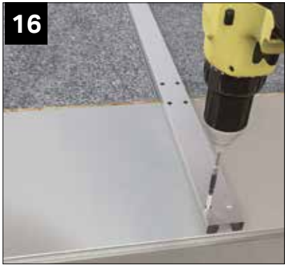
Finally secure the external clips using WPCS020 4.8mm x 38mm self drilling screws provided. NOTE: do not stand on the panels to secure the external clips. Tip: on greater projections secure the clip to the beam (as step 16). Then fit the first row of OSB boarding, this will allow easier access to secure the panel clips further up the roof.
