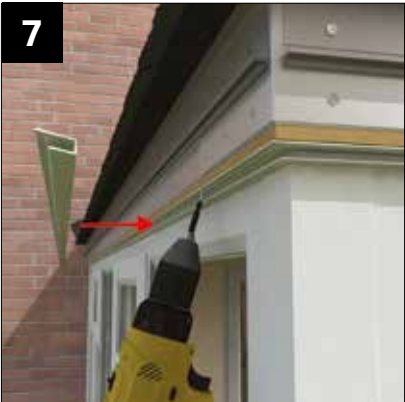
Screw fix PVCu soffit channel into head of window frame or base of OSB board (screws not provided).
