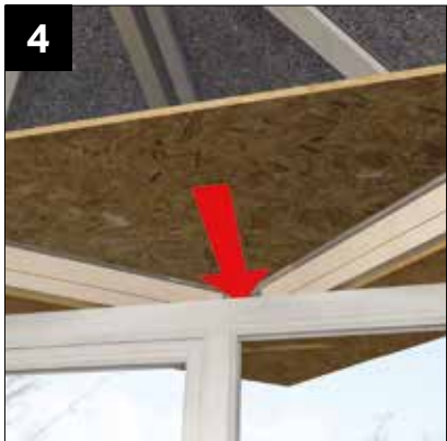
4 Slide into position additional external OSB board.
