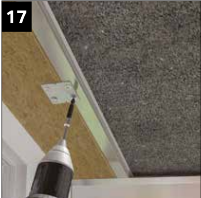
When all external panel clips are installed, fix (at 1 metre centres) using the supplied gable tie-plates WPPC002 using 4 x NRTS050 screws provided.
