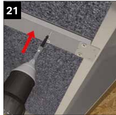
Secure into the panel (at box beam end) as previous image. Again, note method of alternate tightening sequence 22 to 24.
