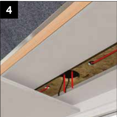
At pitches lower than 17 degrees there is insufficient space on the vertical face to fit the 20mm grommet. Drill 2 holes either side of the light fixing to allow installation of the wires as shown. A 'channel' can be created using 2 narrow strips of plasterboard covered with a top panel.
