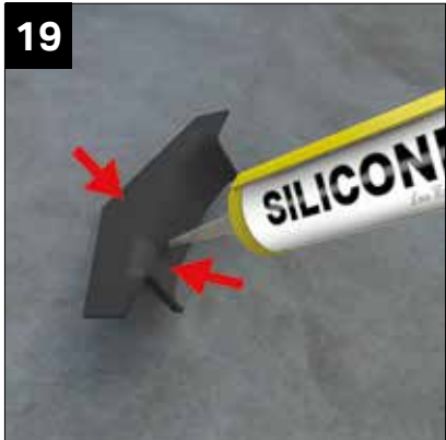
Apply clear low modulus silicone to the faces shown and refit.
