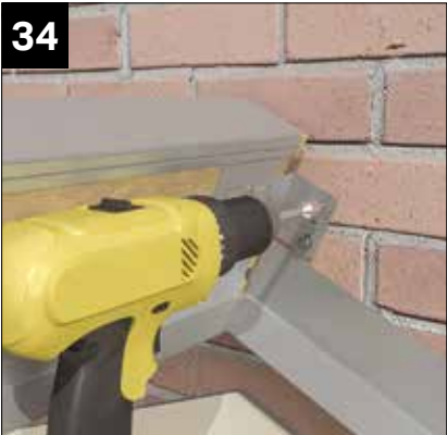
Once ridge is set and level, secure to the host wall using resin anchors suitable for substrate (NOT PROVIDED).
