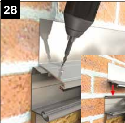
Centralise and fit the half ridge aluminium top capping. Secure using 4.0 x 13 CHAA06 screws provided at 500mm ctrs. Beware: longer screws may penetrate glass.
