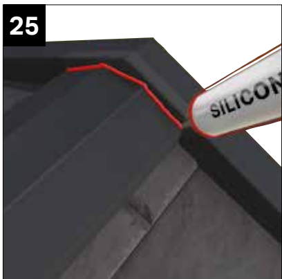
Apply clear low modulus silicone to the joint between the ridge top cap and the dry verge.
